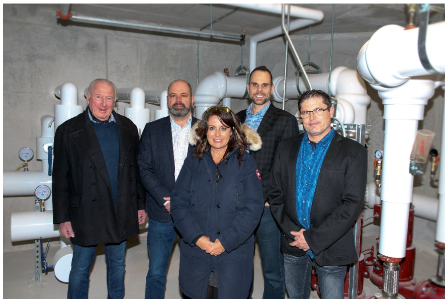
Figure 3.1: Kim, John Blackburn, Michael Williamson and the Divero Energy Team pose with the Geothermal Equipment
