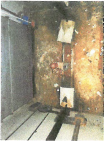
Existing car tops and pit equipment:
