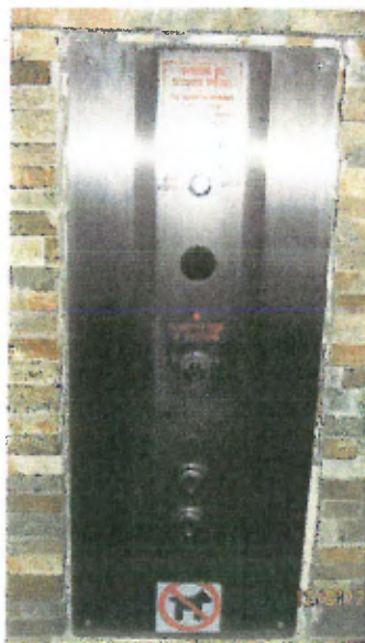
New extended hall station
