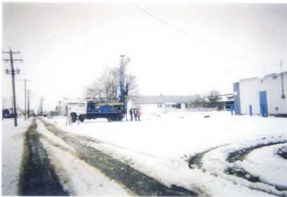
Photo No. 12: May 6, 2002; Phase II Hydrocarbon Environmental Site Assessment Lots 5 & 6, Block 28, Plan 3845 CO; 419 - 10 th Avenue, Carstairs, Alberta Looking North along Alley. Drilling Borehole #7/MW # 3..
