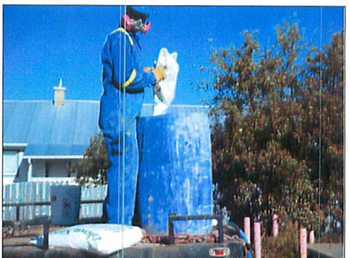
PHOTO 5 View of G&R mixing batch of nutrient water.
