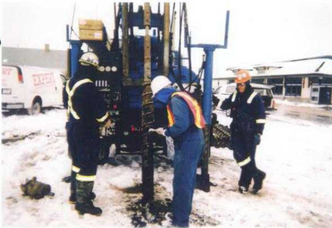
Photo No. 9: May 6, 2002; Phase II Hydrocarbon Environmental Site Assessment Lots 5 & 6, Block 28, Plan 3845 CO; 419 - 10 th Avenue, Carstairs, Alberta Borehole # 2/MW #1. View of PES Staff Collecting Soil Samples.
