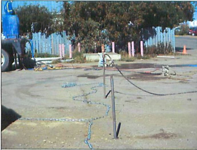
PHOTO 6 View of injection points facing north.
