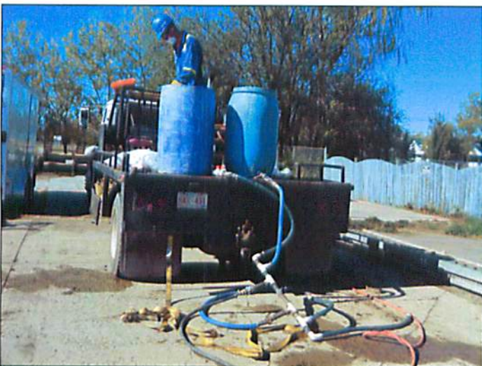
PHOTO 4 View of nutrient mixing system.
