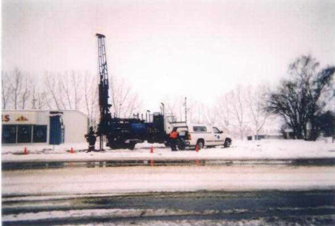
Photo No. 7: May 6, 2002; Phase II Hydrocarbon Environmental Site Assessment Lots 5 & 6, Block 28, Plan 3845 CO; 419 - 10 th Avenue, Carstairs, Alberta Looking West. Drilling Borehole #1.
