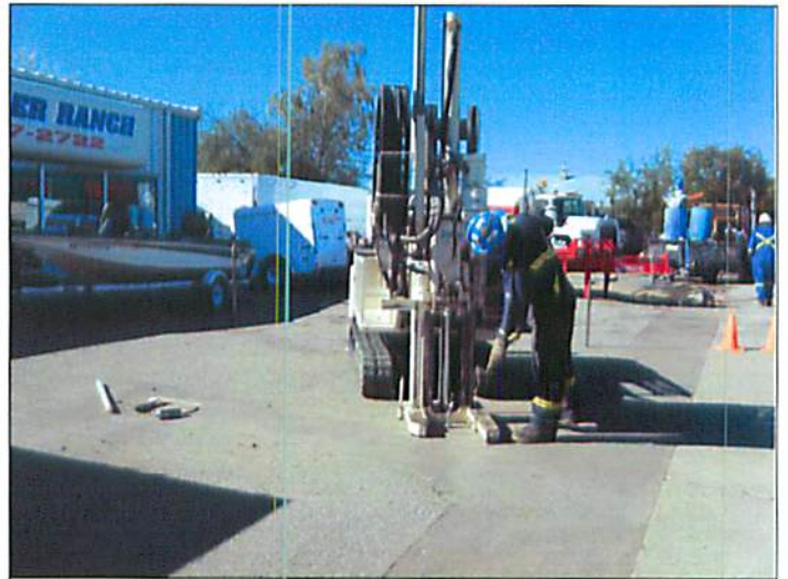
PHOTO 7 View of direct push rig installing injection well.
