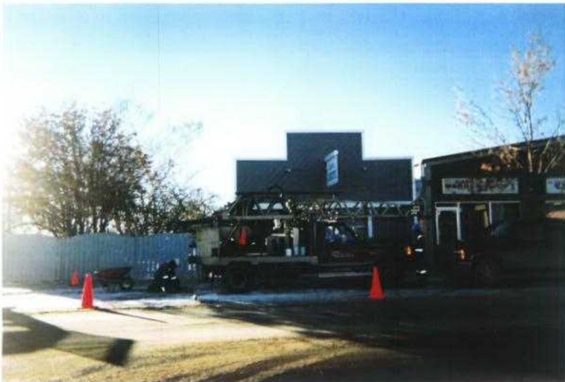
Photo No. 14 January 15 & 16, 2003; Phase III: Hydrocarbon ESA-Delineation Lots 5 & 6, Block 28, Plan 3845 CO; 419 - 10 Avenue, Carstairs, Alberta Looking West. Borehole #24. Finishing The Borehole Surface.
