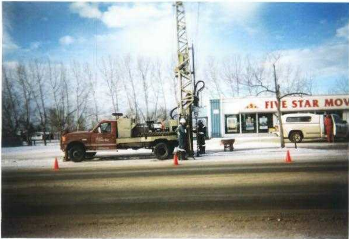
Photo No. 11 January 15 & 16, 2003; Phase III: Hydrocarbon ESA-Delineation Lots 5 & 6, Block 28, Plan 3845 CO; 419 - 10 Avenue, Carstairs, Alberta Looking West. Drilling Borehole #19.
