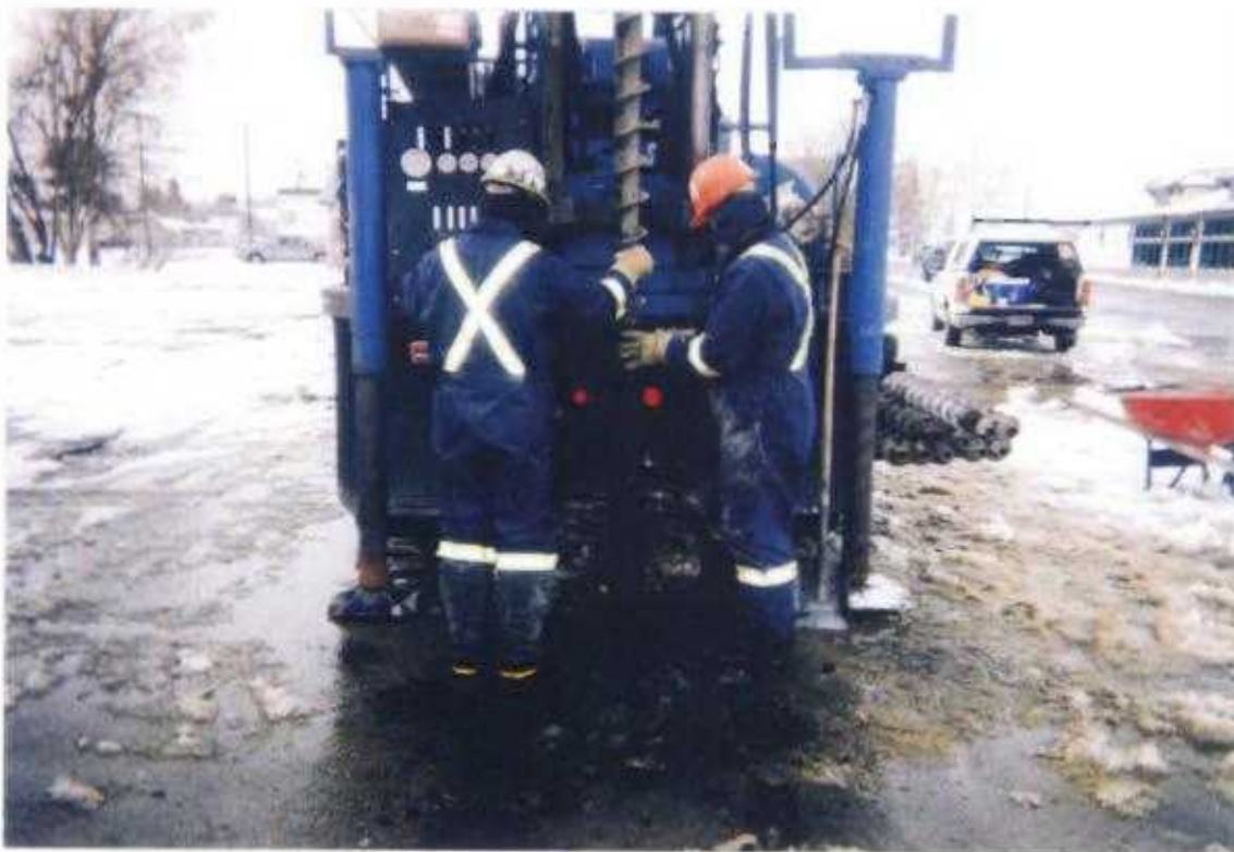
Photo No. 8: May 6, 2002; Phase II Hydrocarbon Environmental Site Assessment Lots 5 & 6, Block 28, Plan 3845 CO; 419 - 10 th Avenue, Carstairs, Alberta Looking North. Drilling Borehole #2/MW #1. View of First Auger Flyte. Note: Heavy Black Staining.
